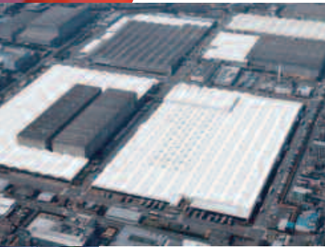
Nissan Building—After coating
